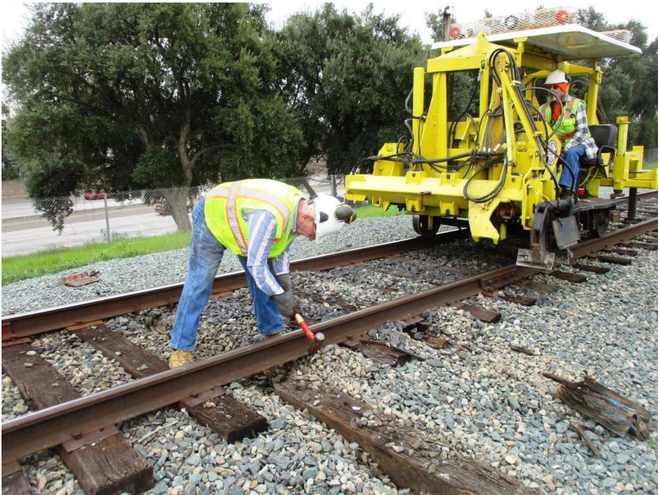
Clem removes rail-anchors near the extracted tie
