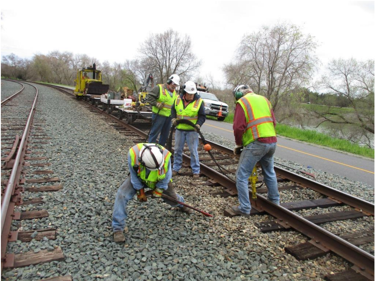
Joe nips-up the tie, Bill and Art handle the hoses as Steve drives a spike with the hydraulic spike-driver
