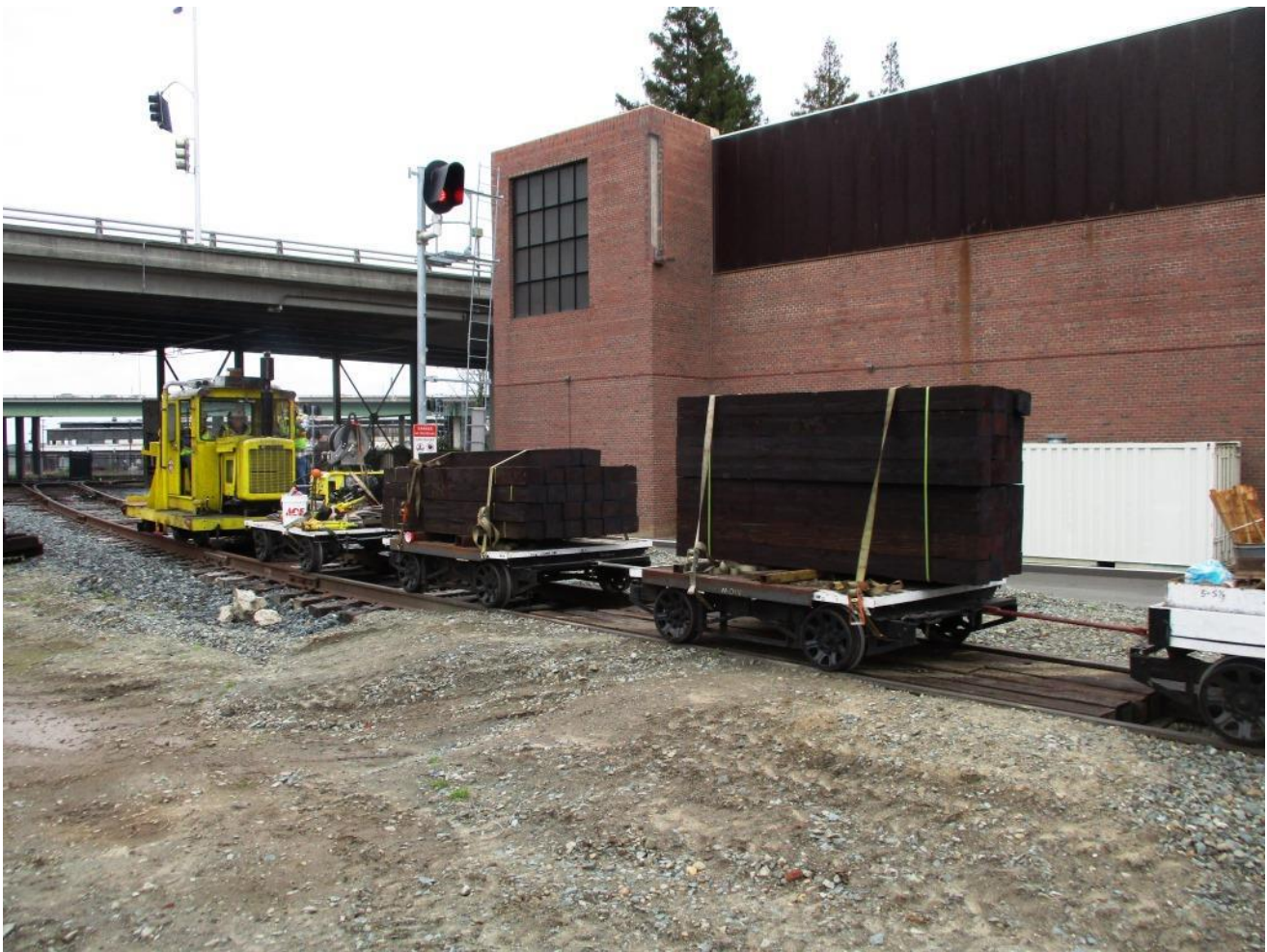
With ties now loaded on flatcars, Bill in the Kalamazoo shoves the MOW work-track across the UP Main
