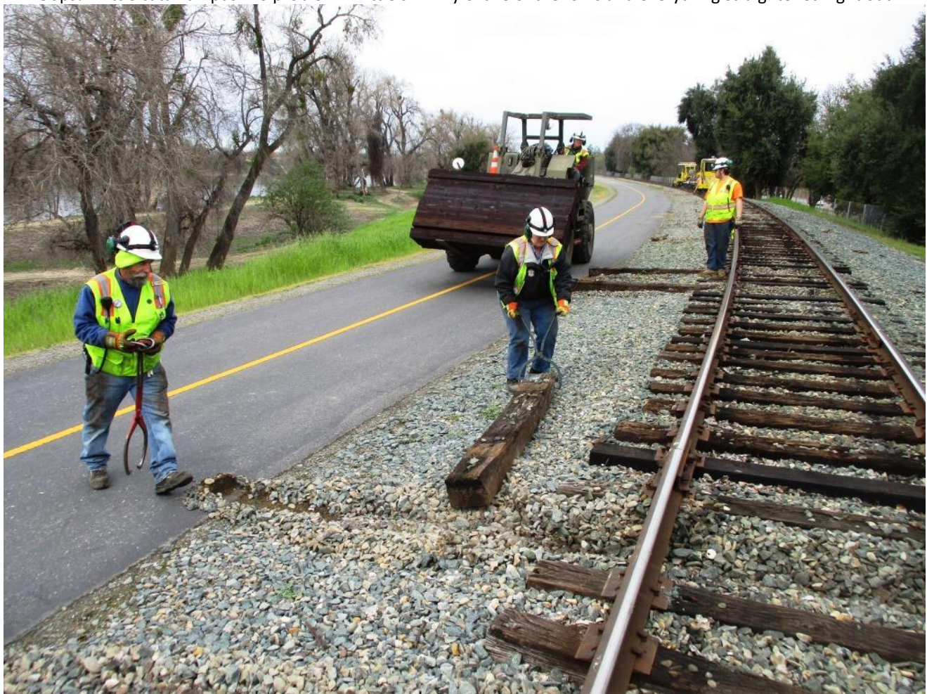
Heather and Joe move old ties out of the way so that Steve on GM2 can come in to distribute new ties
