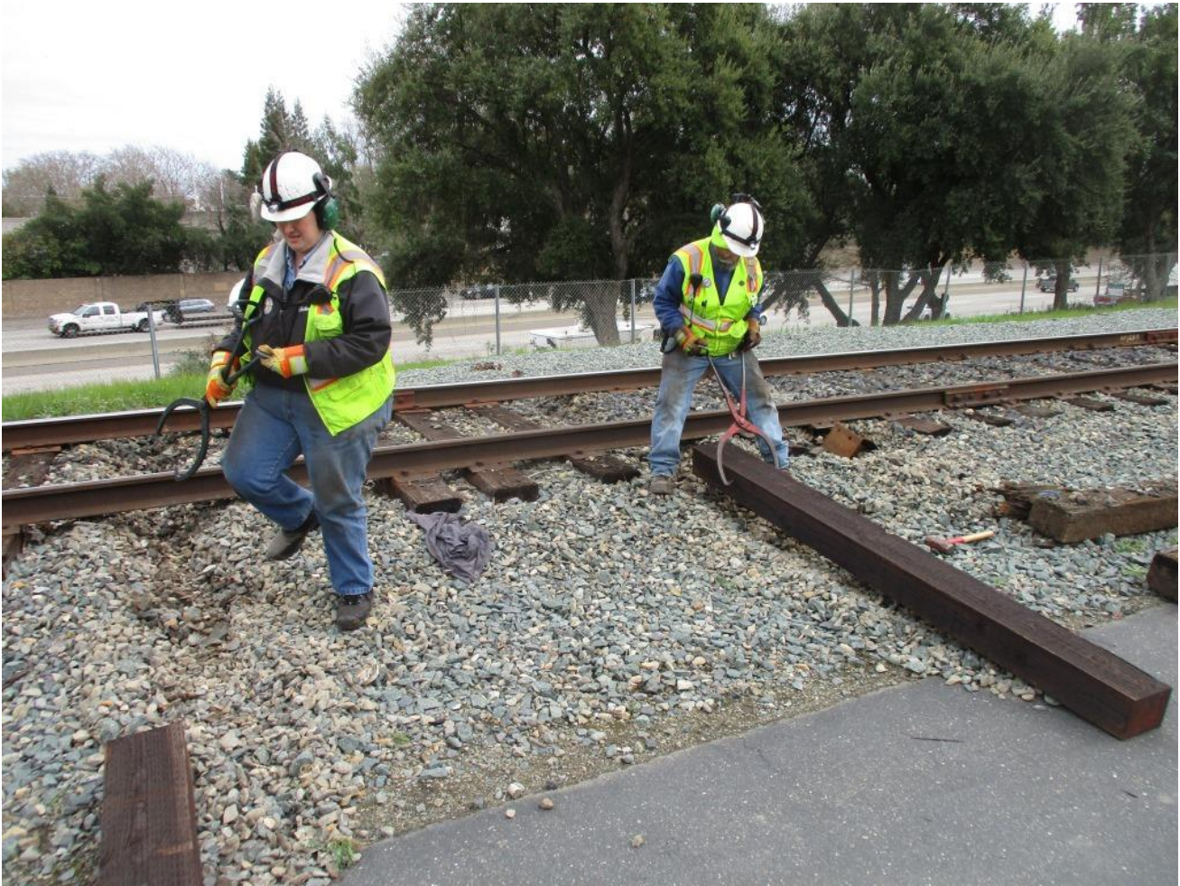
Heather and Joe get the tie-ends under the base of the rail
