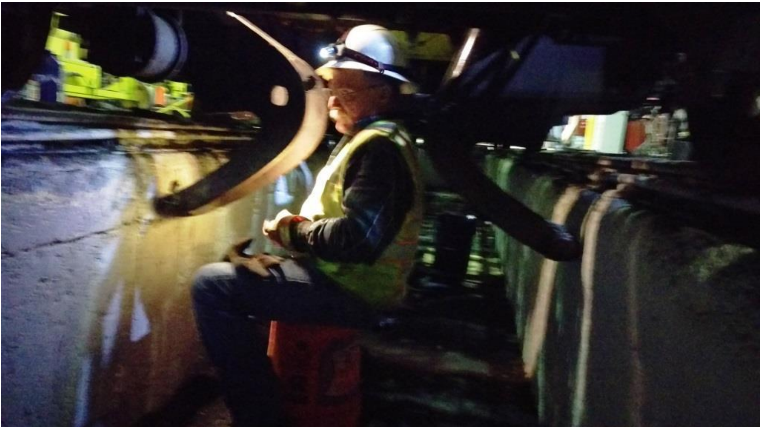
Deep within the "pit of despair," Mike H. begins reattaching the cylinder
