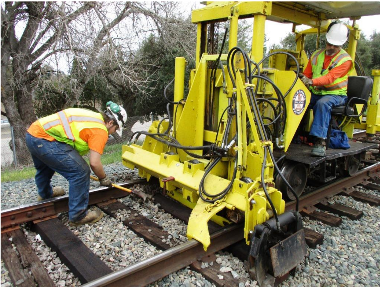
As Ed uses the 125's track-jacks, Chris prepares to insert a tie-plate between the base of the rail and the tie
