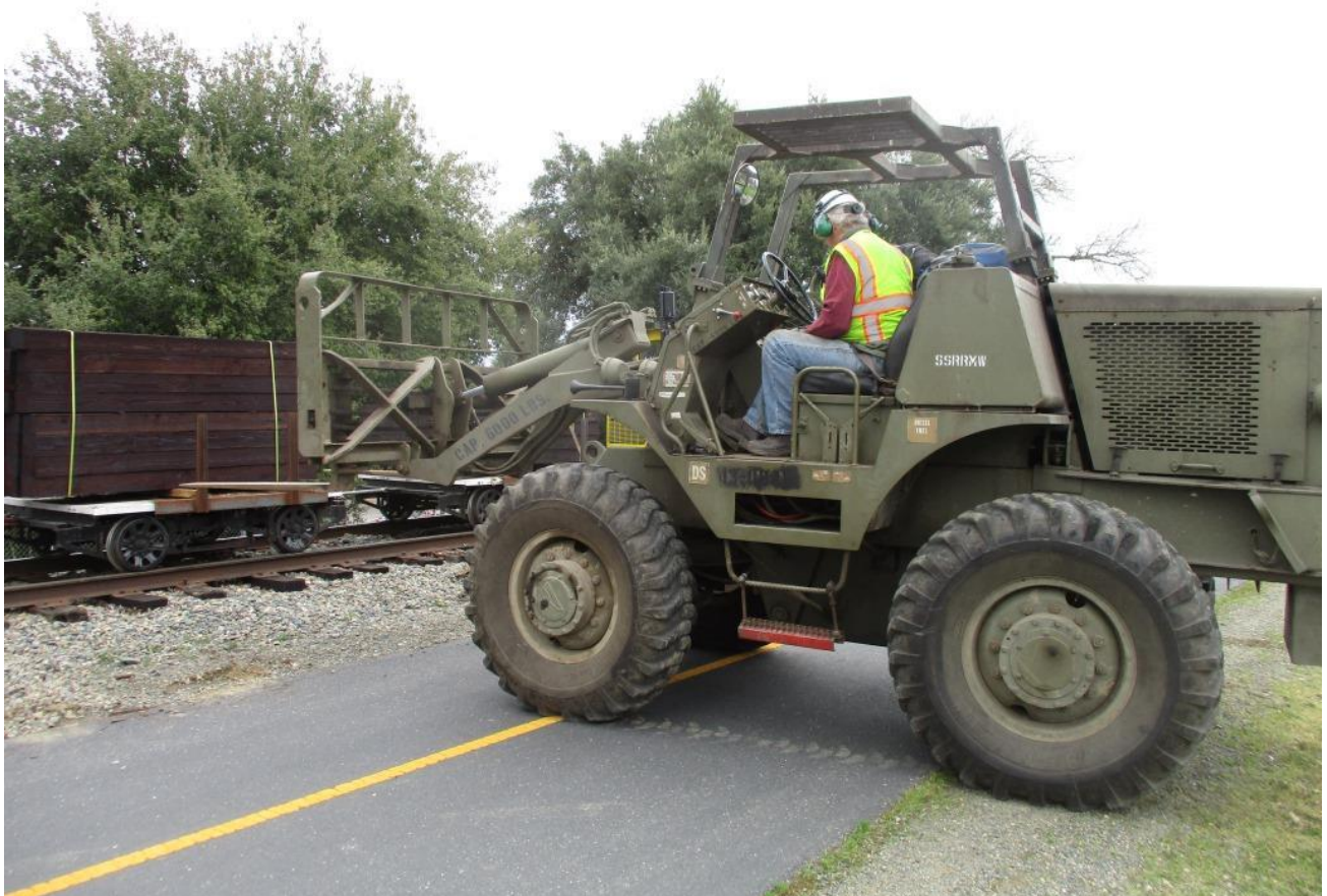
Steve returns to the work-site to grab the bundle of ties for distribution along line
