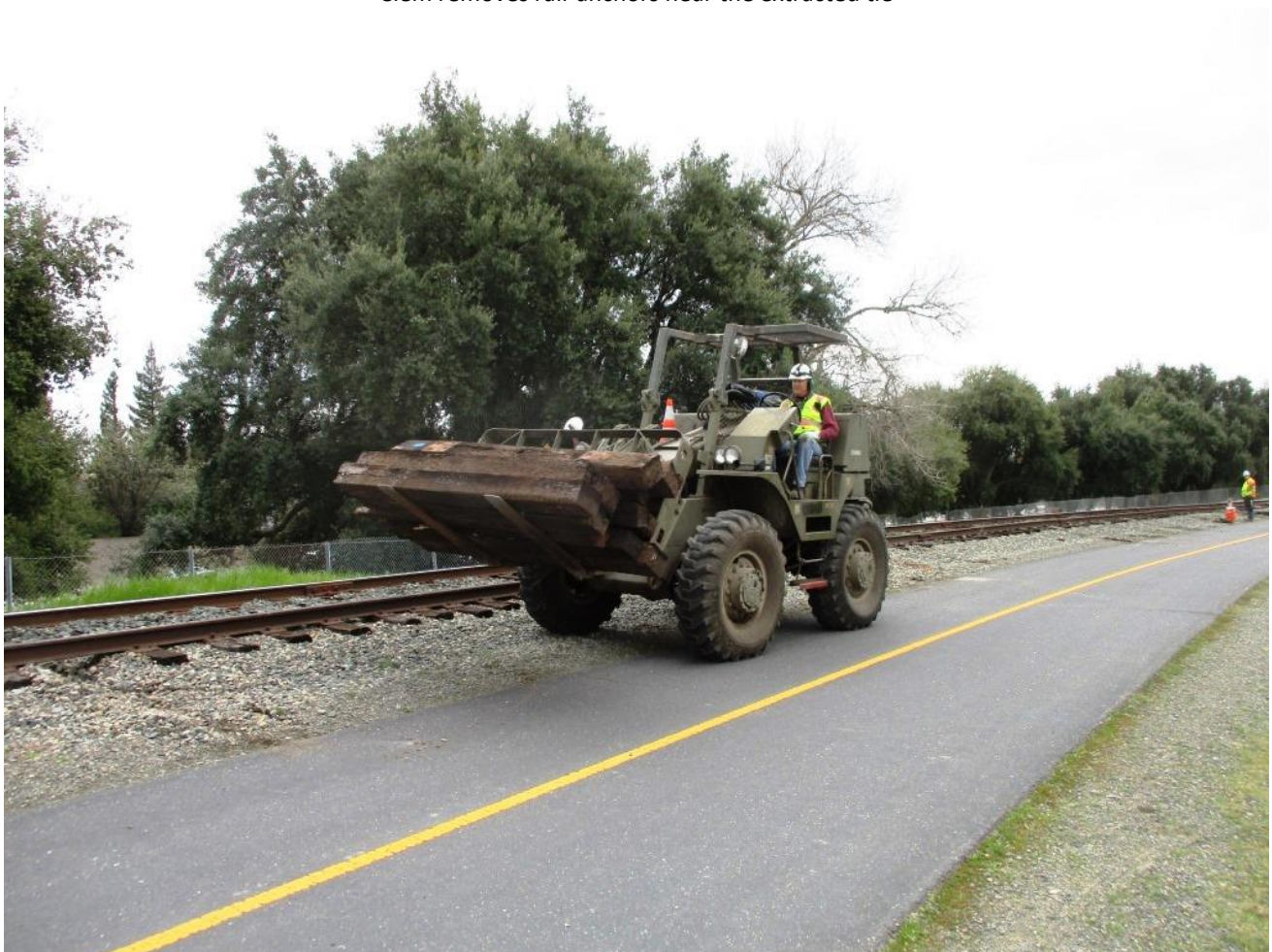
Steve on GM2 takes those old rotten ties to Setzer for disposal. A shop forklift certainly couldn't do this kind of work
