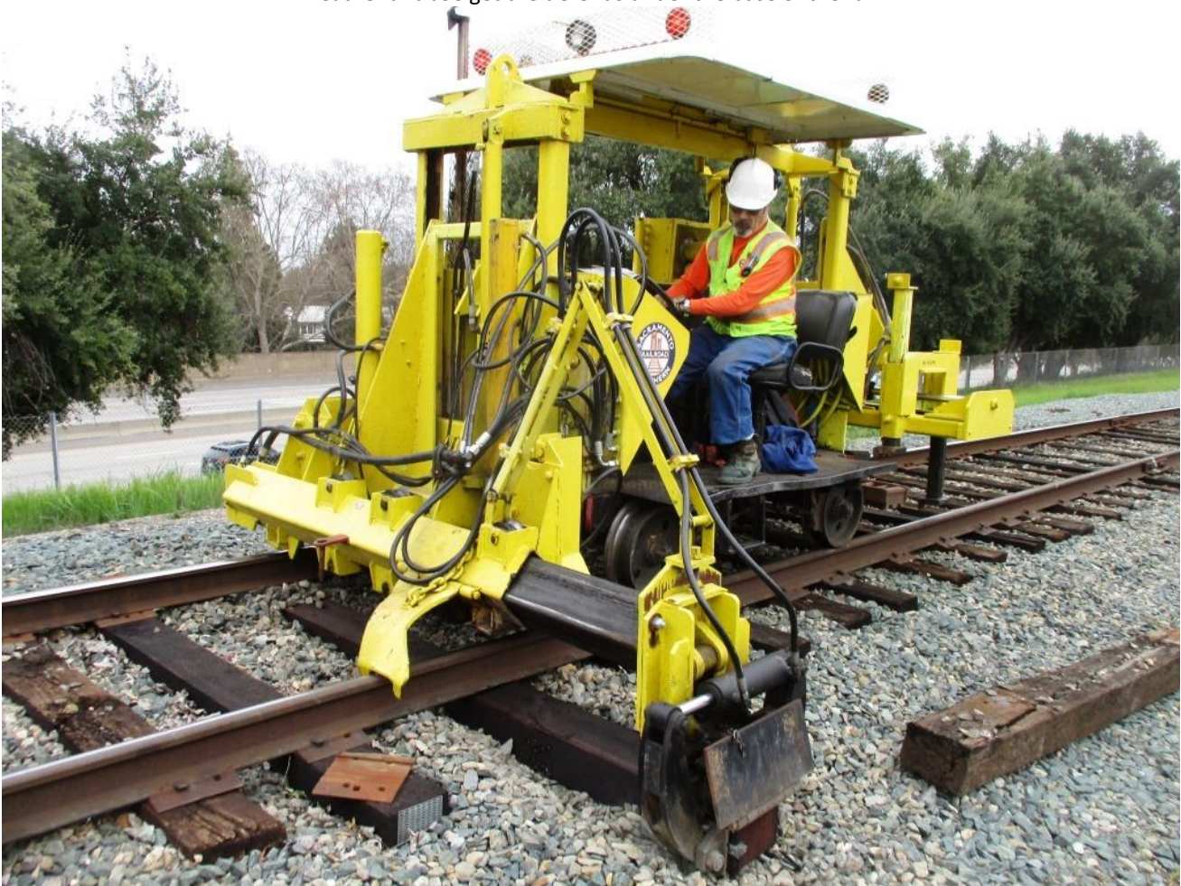
Ed pulls a new tie into place
