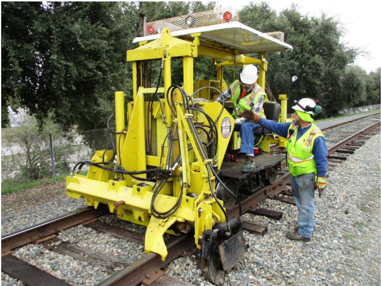
Joe trains Ed on the operation of the Jackson 125 tie-exchanger
