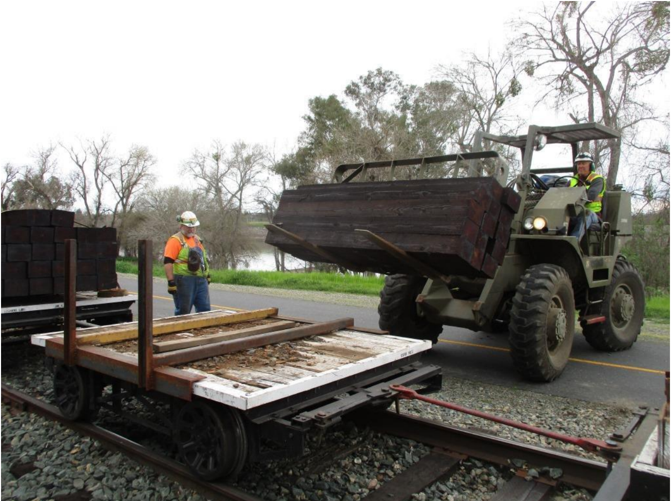
Steve brings in the remaining new ties and re-loads them on the flatcar as the Team prepares to head back to town
