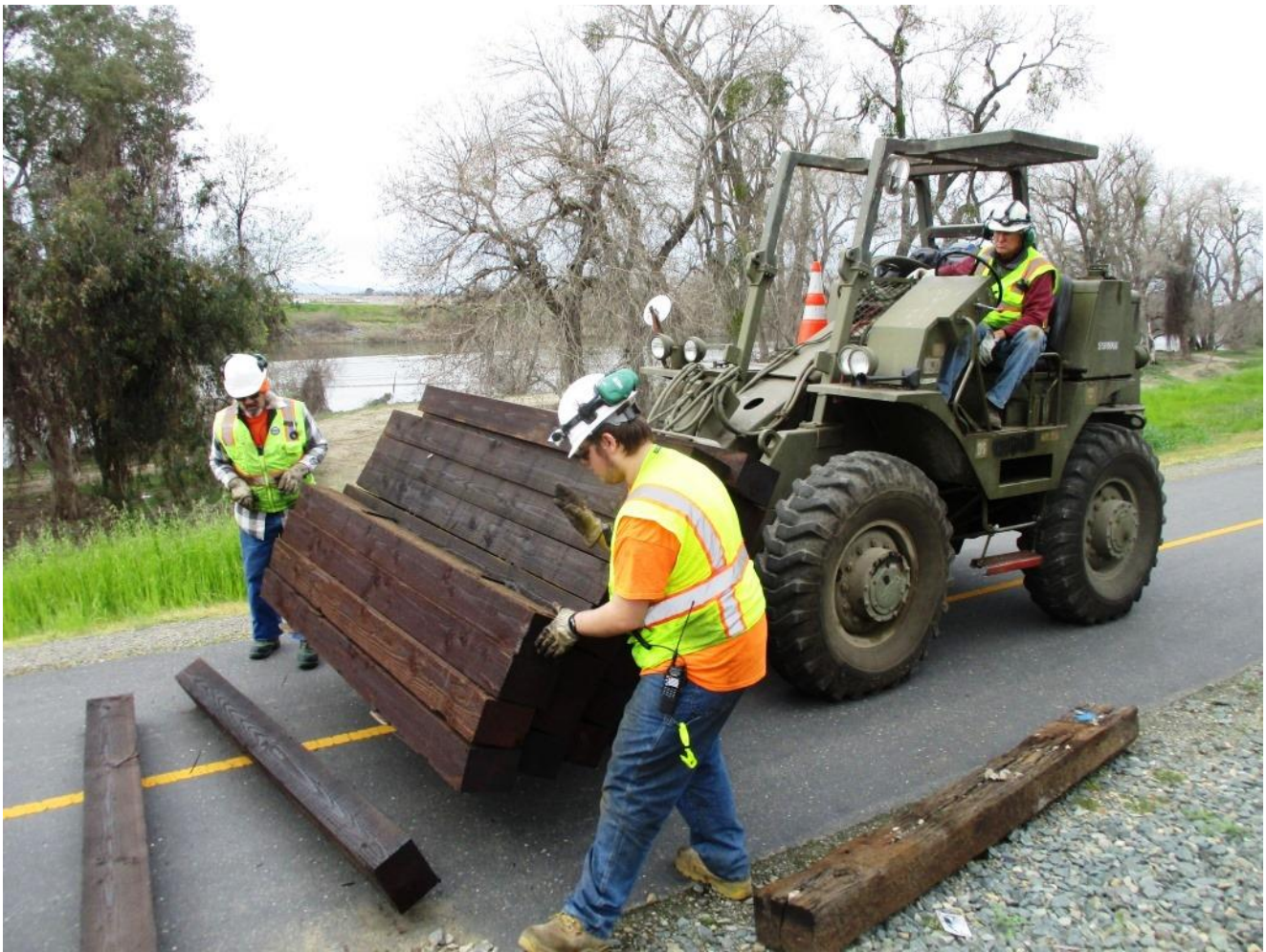
Ed and Chris roll new ties off the bundle...
