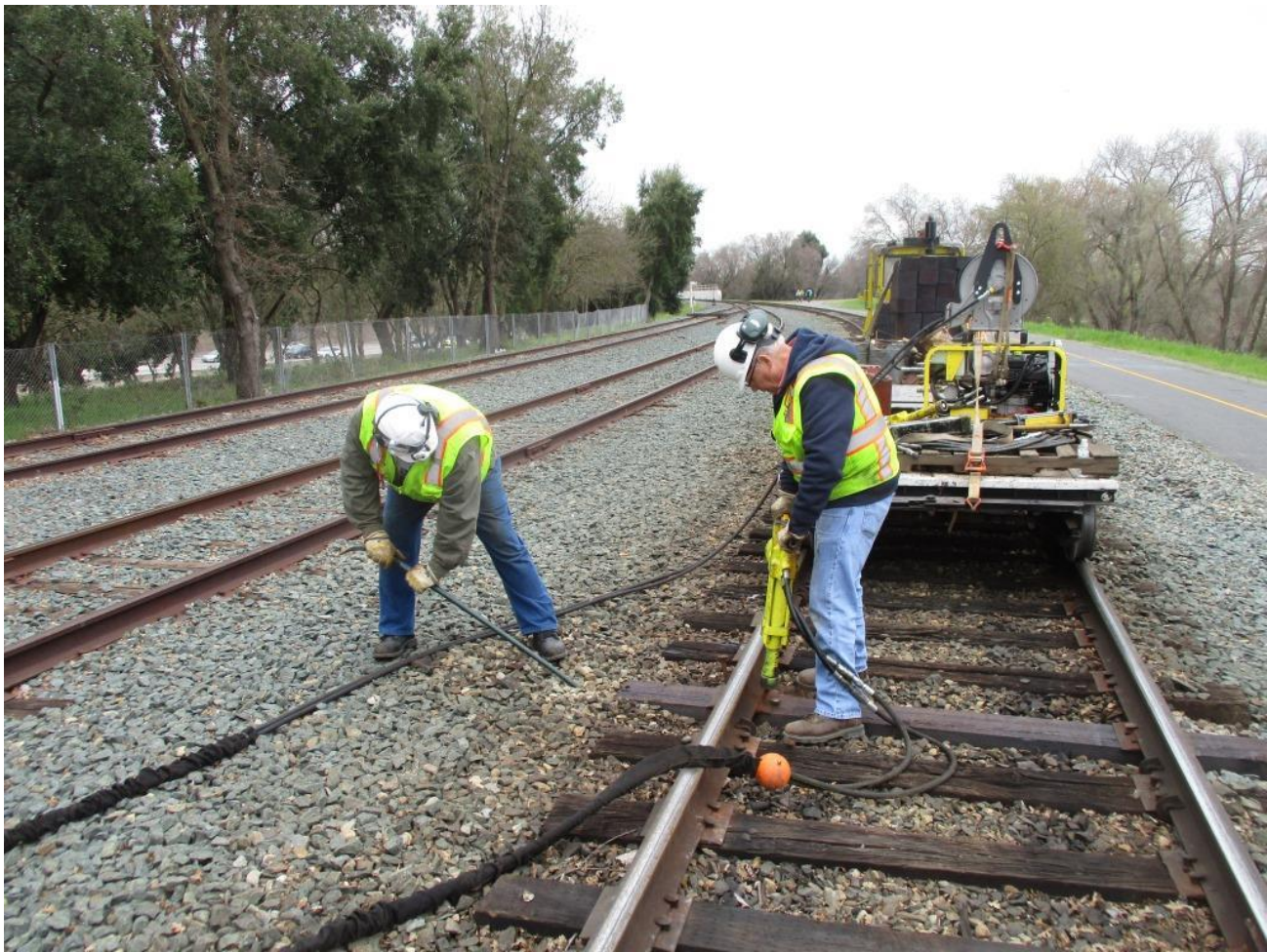
Art nips-up the ties as Bill drives spikes with the hydraulic spike-driver
