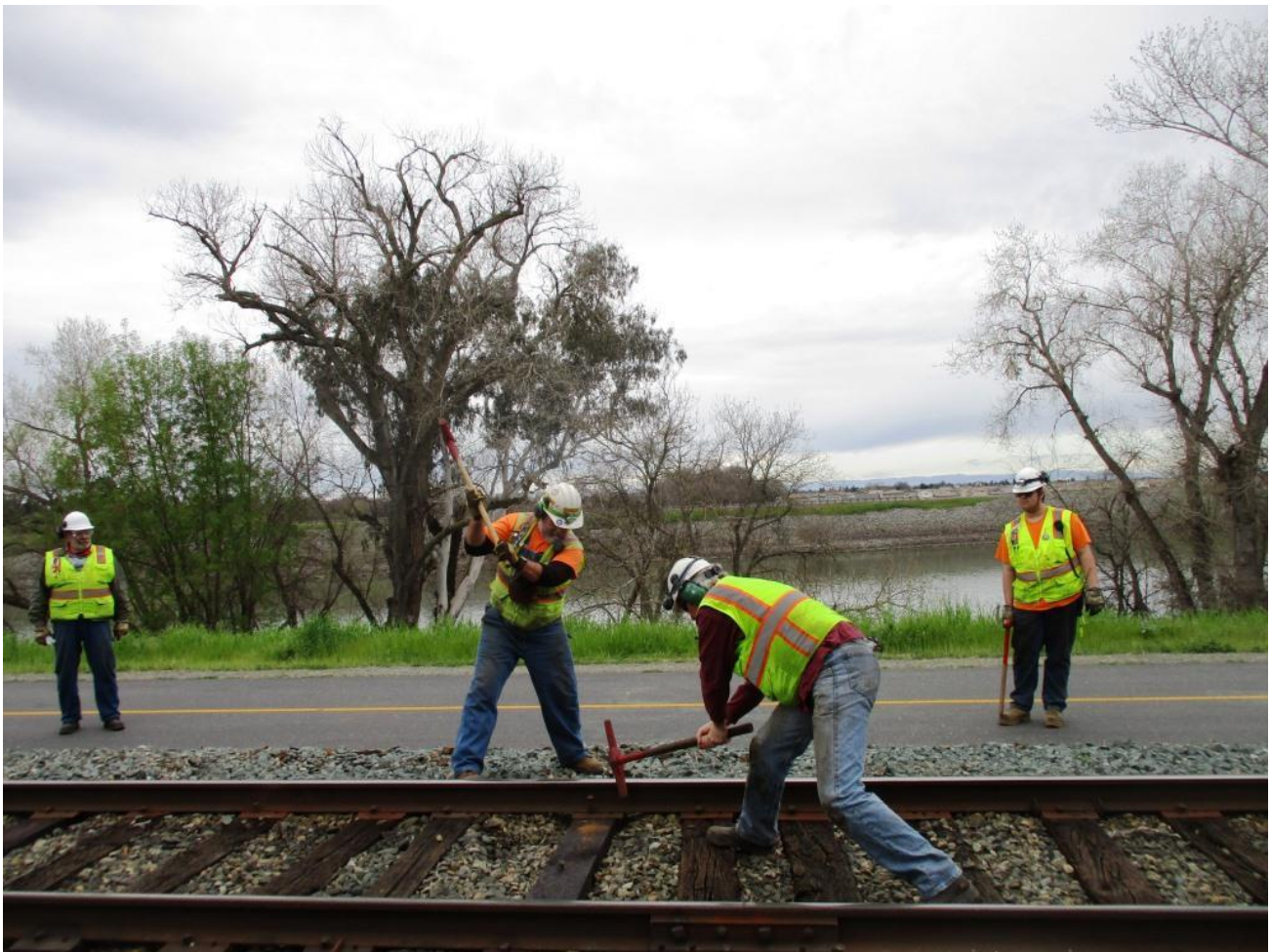
They're at it again! Mike F. and Steve interpret old fashion track-gang railroading with their tandem spike driving technique
