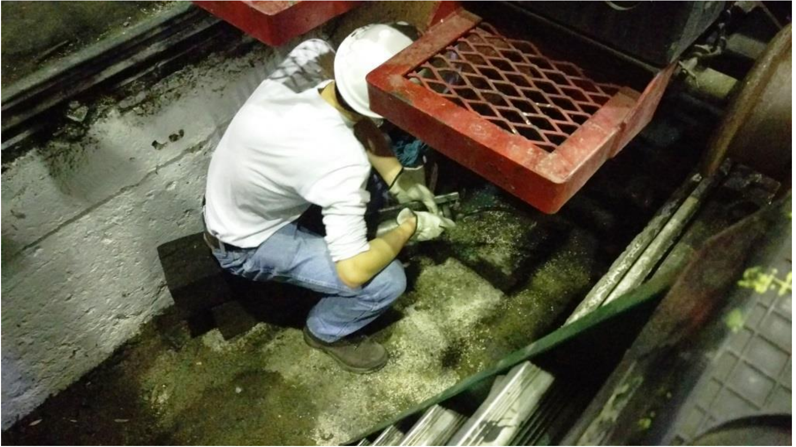
Jack descends into the pit under the shear to assist Mike H.
