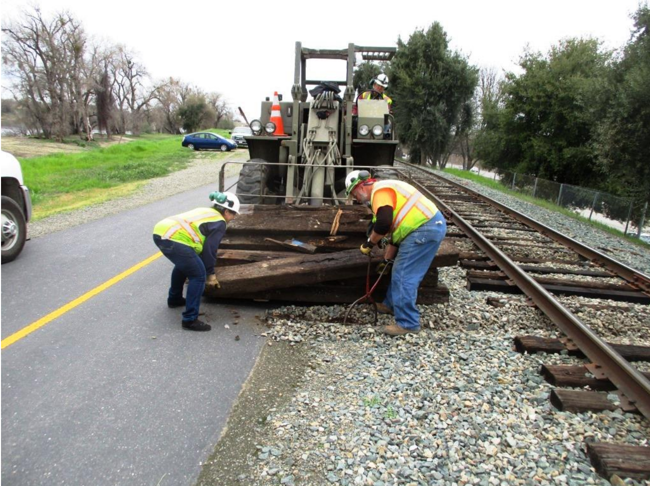
As rotten ties come out, Steve on GM2 collects them for disposal. Pam and Mike F. help scoop them onto the forks
