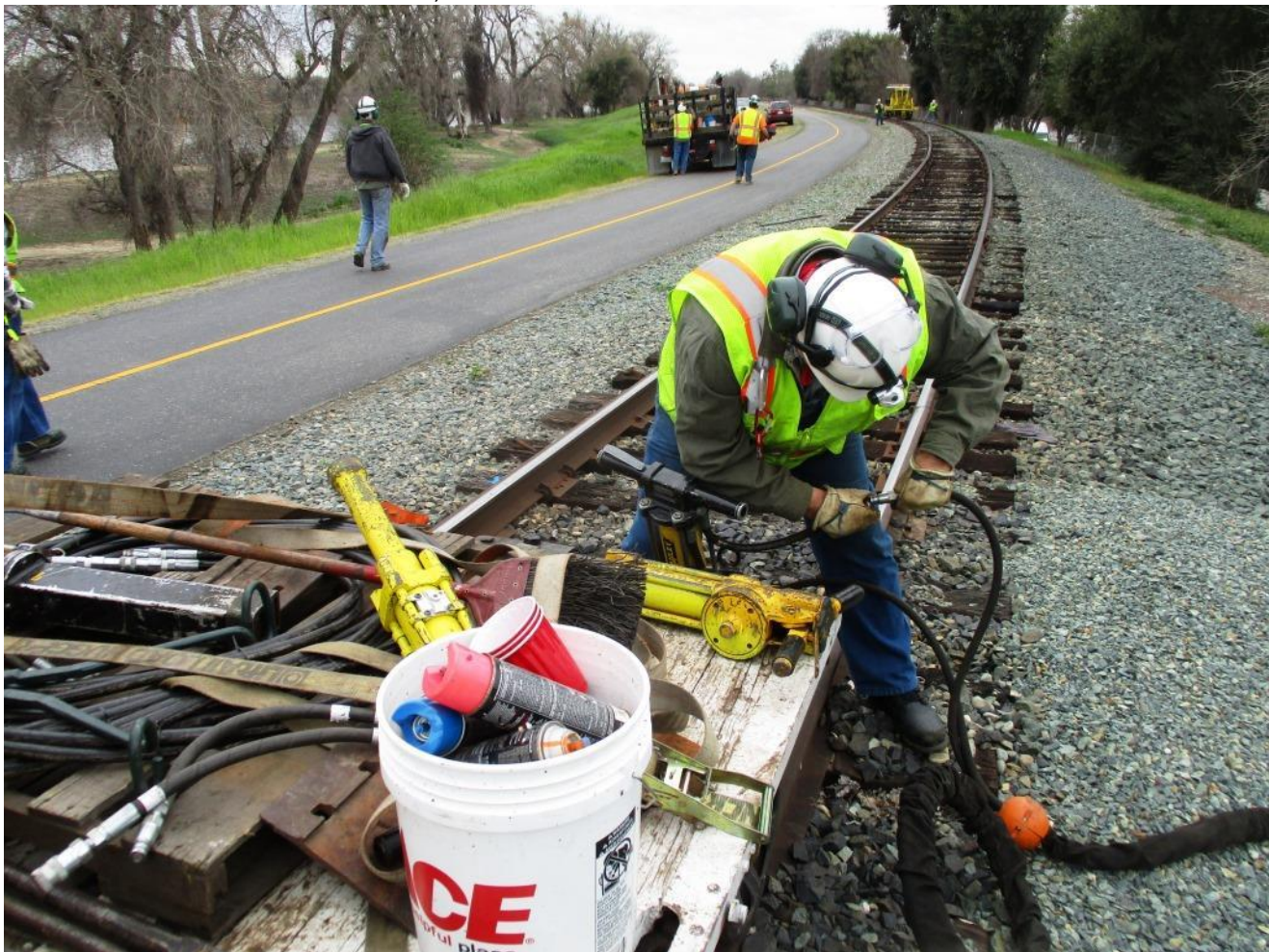
Art connects the hydraulic hoses to the hydraulic spike-puller
