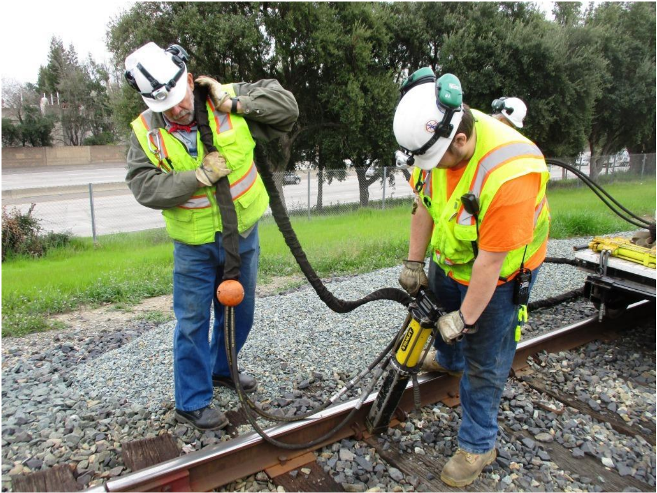
Art handles the hoses as Chris pulls spikes with the hydraulic spike-puller
