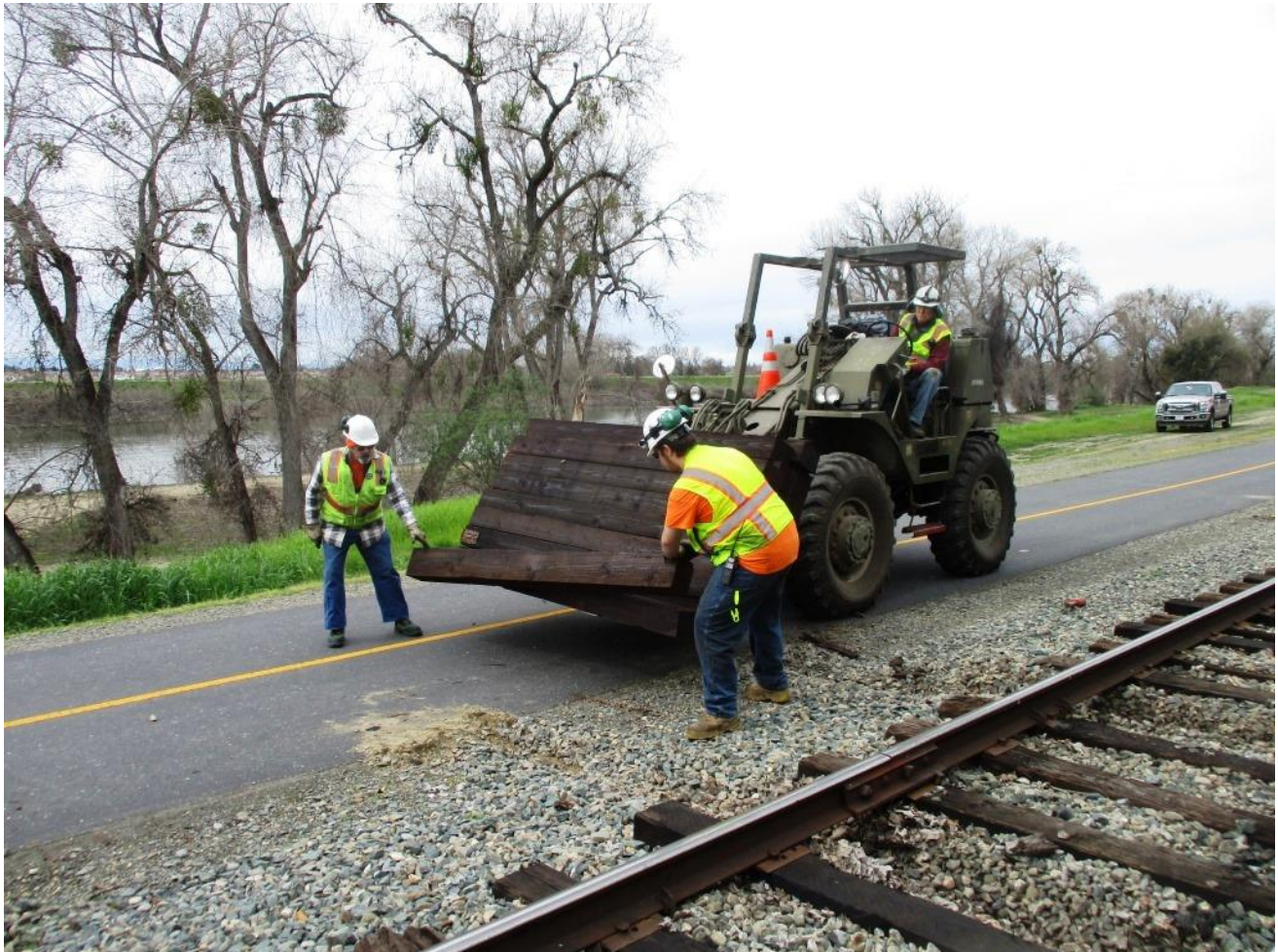
...Next to the cribs where they will be inserted
